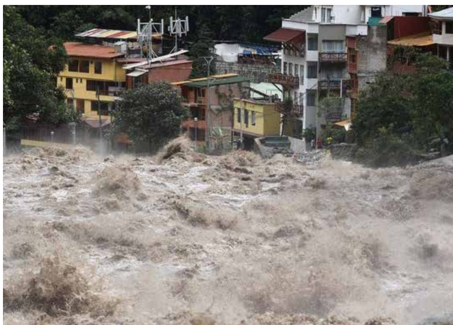
Severe flooding of the Vilcanuta River in Macchu Pichu, Peru. Source: Ross, 2016
