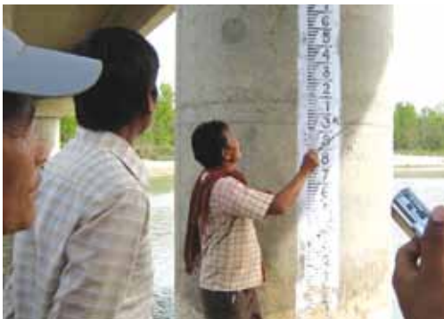
Photo 7: Gauge painted on bridge pillar
